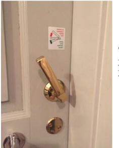
These were the niftiest door handles in Sweden. To lock the door you lift up and the handle stays put. To unlock and open the door you just push down.
