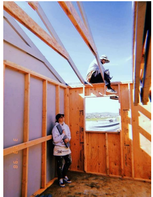
On the build site :)
